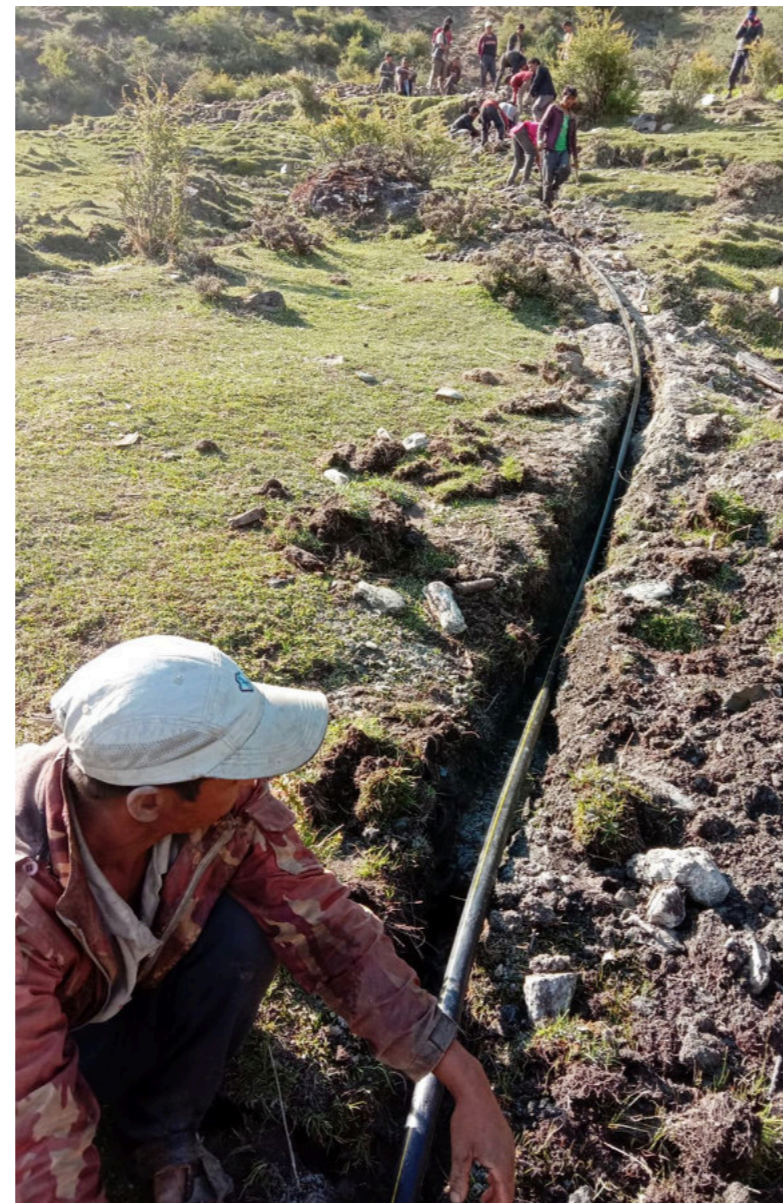
Conducting maintenance and repair of drinking water system in Dolpa.
