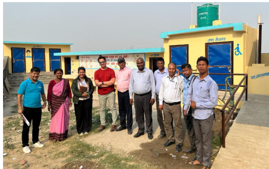
WASH plan implementation at Shree Secondary School, Chhata Pipra
