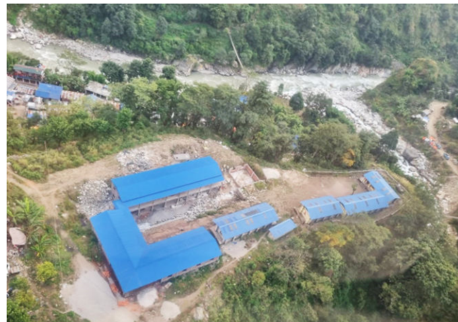
Dharche Community Hospital
